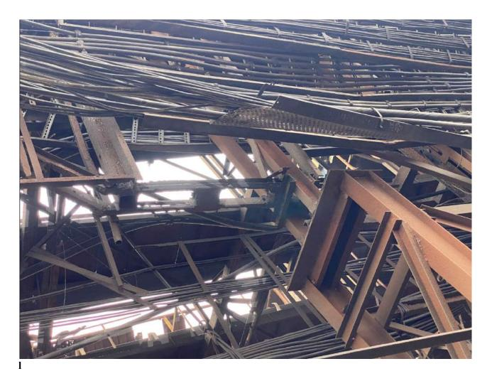
In past strengthening or repairing of the above conveyors structure has been done, but now it is beyond repairable and its post dislocated from concrete foundation. Hence it is recommended to take up the work of Renovation/Upgradation/Modification of Belt Conveyor 10A/B/C with allied works on urgent basis in CHPA, so that bunkering conveyor stream BC 10A/B/C will run sustainable capacity.
