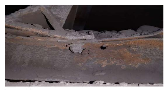
The rusted deck module needs immediate complete replacement with providing proper angle support underneath and painting with anticorrosive paint. In past strengthening or repairing of these damaged stinger channel /angle post has been done, but now it is beyond repairable and its angle post dislocated from concrete foundation.
