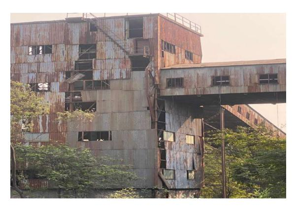
To address above, Transfer point vibrations analysis along with structural audit will be required and necessary modification & modernization of Transfer Pontstructure is recommended. The dust emission is occurred in Transfer Point during transportation of coal. Transfer Pontstructure is to be covered with new upgraded size and type of sheet for longer service life with proper enclosure to avoid dust ingress in atmosphere.
