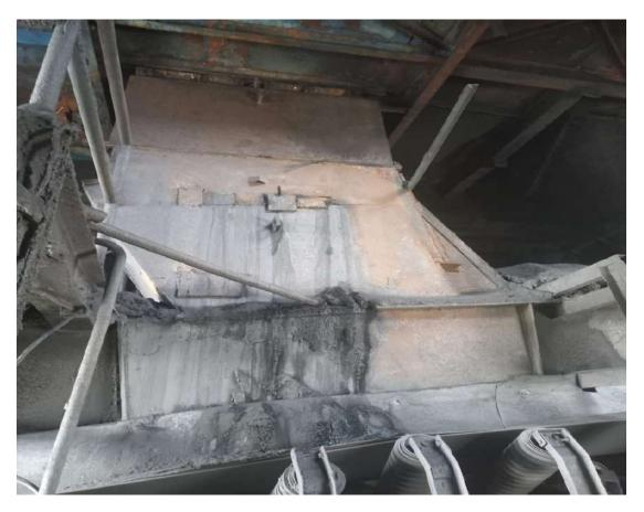
Due to repeated patching & other work, these chutes are beyond repairable and need replacement on urgent basis to avoid secondary damages to costly conveyor system and to avoid hampering the unloading of 'N' box wagons. Hence to avoid coal spillage and to ensure smooth operation of coal handling plant, timely replacement of these chutes plates with suitable wear plates of sufficient hardness & suitable material composition is required as per wear pattern & coal flow trajectory.
